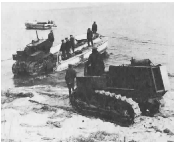
Forty-five foot artillery lighter (Artillery Lighter "B") unloading a 5-ton tractor at Quantico in 1935. Troop Barge "A" is shown in the background.
