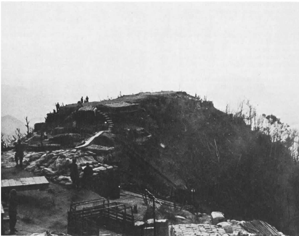
Fire Support Base of the 3d Marine Division near the Rock Pile in January 1969. (USMC Photo #A192512).
